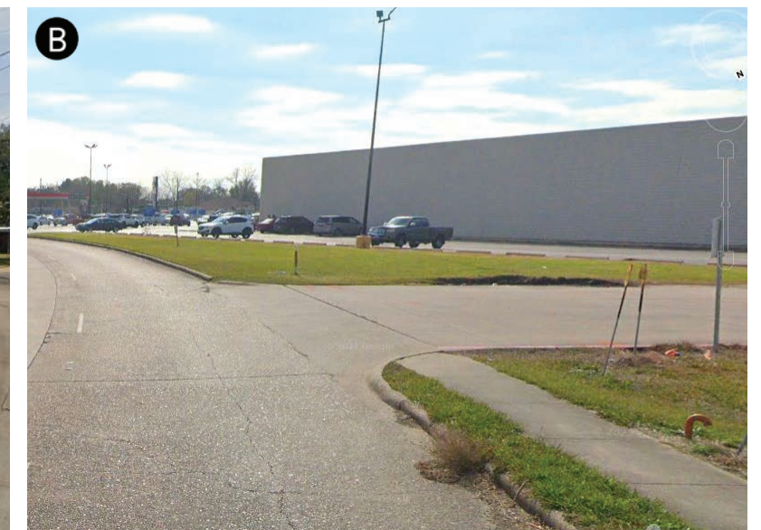
Figure 13. Missing Sidewalk Connection to Grocery Store
