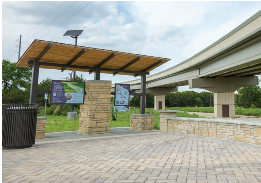
Example of wayfinding and placemaking at a trailhead
