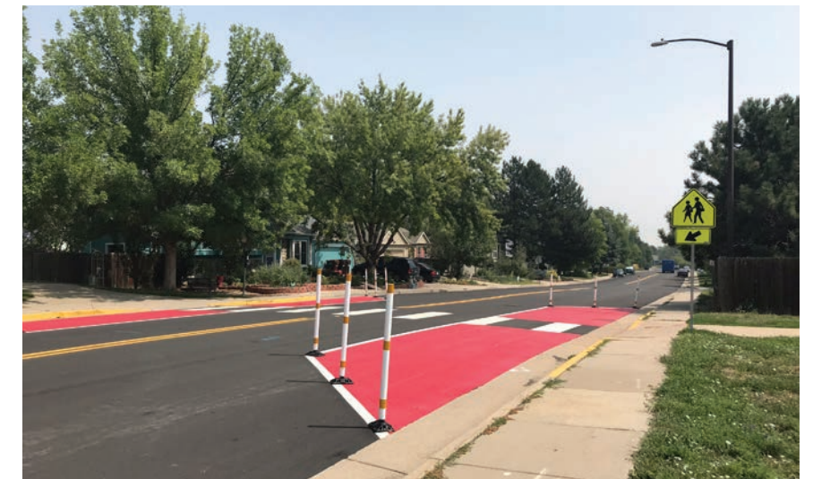
Example of reduced crossing distance for a trail across a neighborhood street
