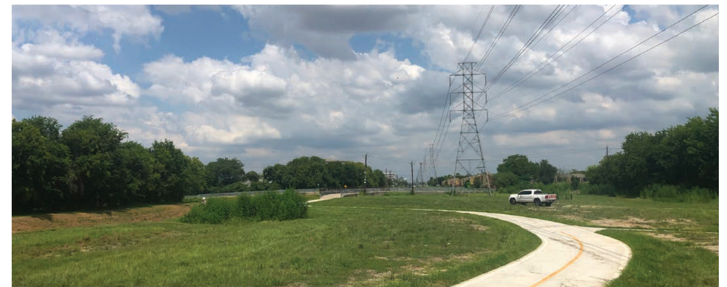
Example of a trail within a utility easement in Harris County
