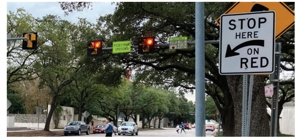
Example of a midblock crossing with HAWK signal
