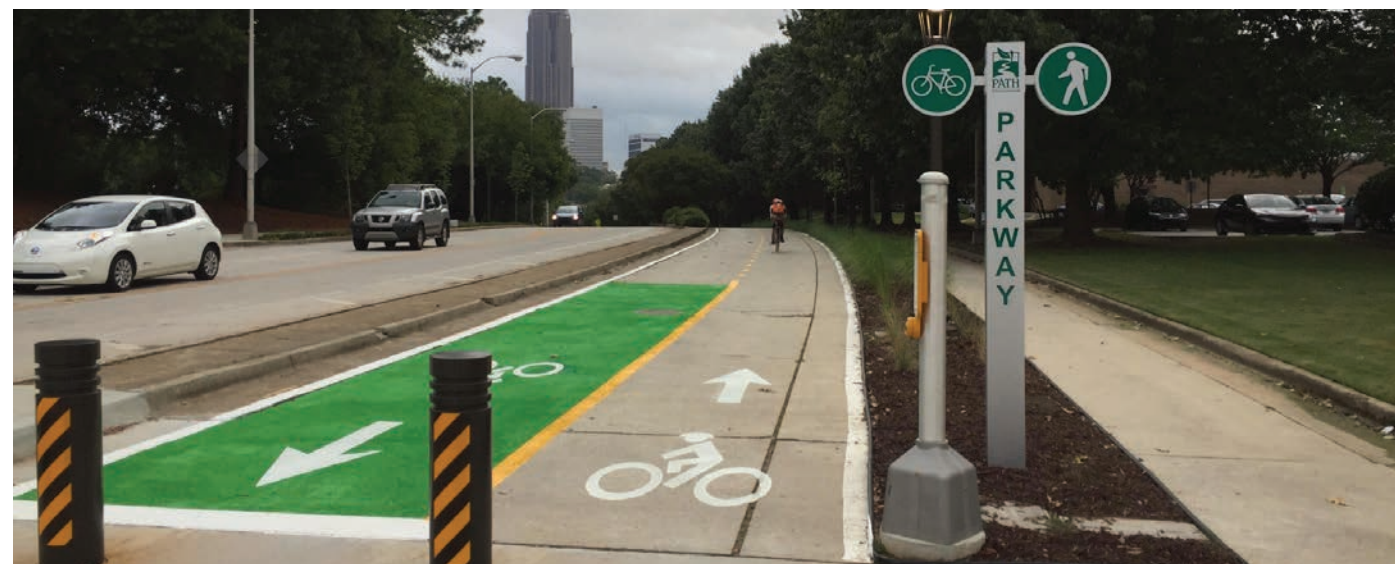
Example of a separated bikeway and pedestrian path with center buffer from Georgia Tech University campus
