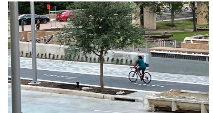
Bagby Street bikeway under construction in Harris County
